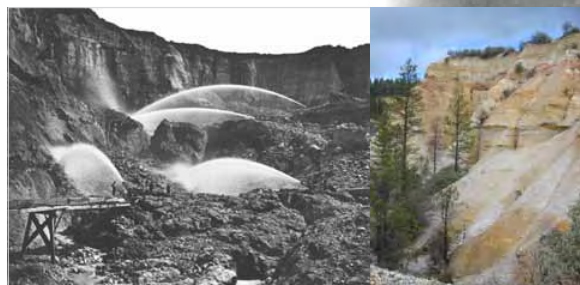
The Malakoff Diggins Mine Pit - Then and Now: Hydraulic mining monitors were used to direct powerful streams of water to wash down hillsides in search of gold bearing gravels. Seven monitors ran day and night and large amounts of mercury were used to extract gold from the resulting slurry. Today, the steep walls left by the mine continue to erode, and in large rainstorms as much as a ton of sediment can be carried downstream.
